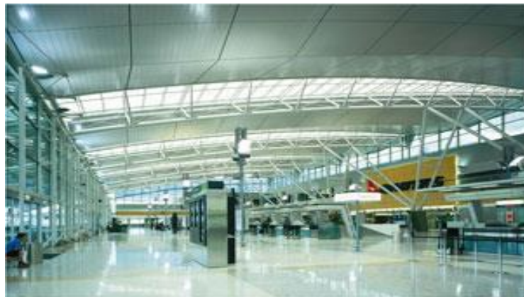
Gambar II.4 Stressbar ties, Qantas Arrivals/Departure Hall, Sydney Airport
