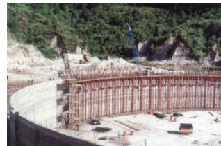
Gambar II.15 Slipform for deep tank, Porsea, North Sumatra, Indonesia
