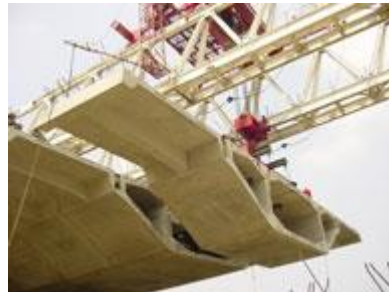
Gambar II.20 Precast segmental balanced cantilever erection with overhead launching gantry Pasupati Project, Bandung, Indonesia
