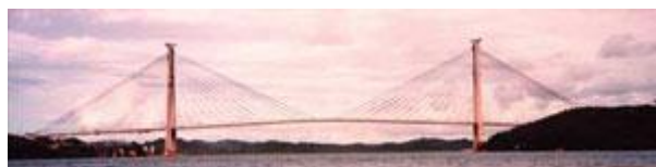
Gambar II.17 Batam-Tonton Bridge with 350m main span, Indonesia
