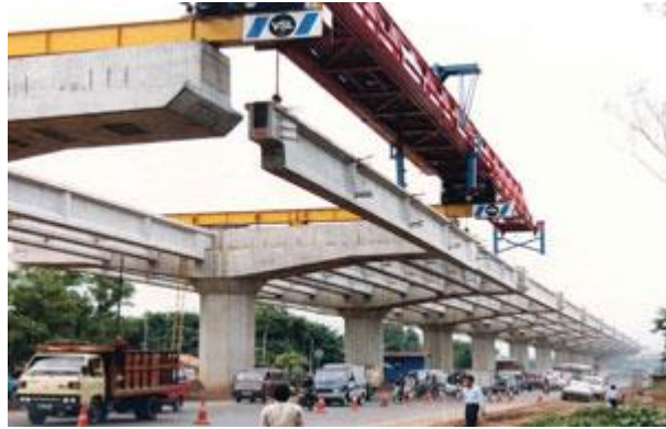
Gambar II.21 Precast girder lifting with overhead launching gantry. Toll road project, Jakarta, Indonesia
