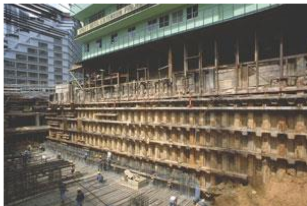
Gambar II.6 Temporary ground anchor, Hyatt Hotel, Jakarta, Indonesia
