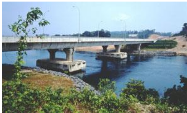
Gambar II.3 Post-tensioned bridge , Bareleng, Indonesia
