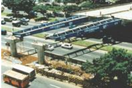
Gambar II. 23 Launching noses crossing over traffic Sudirman flyover, Jakarta, Indonesia
