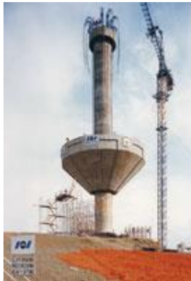
Gambar II.10 Lifting of concrete water tank Karawang, Indonesia
