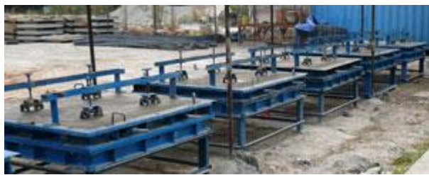
Gambar II.8 Panel precasting, Semplak Project, Indonesia
