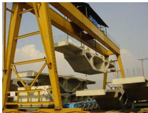
Gambar II.12 Segment lifting at stockyard, Bandung, Indonesia
