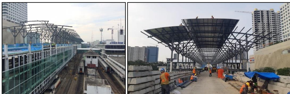
Progress Pekerjaan Saat Bulan September 2018
