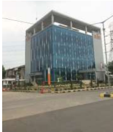
Gambar 3. 5 Dokumentasi Survey Financial Center
